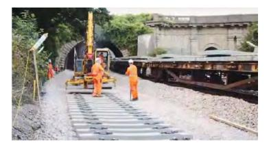
Figure 5-26 Sleeper laying
