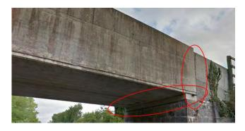
Figure 5-390 Joints to be demolished at abutment
