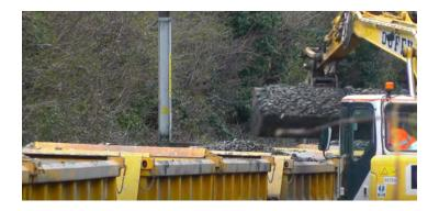
Figure 5-15 Ballast removal
