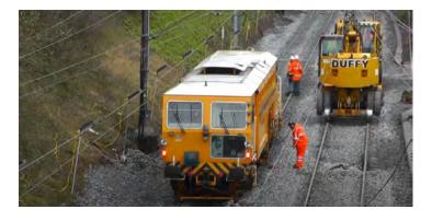
Figure 5-22 Ballast tamping
