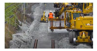
Figure 5-19 Track panel installation
