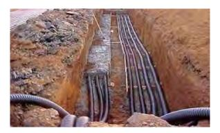
Figure 5-63 Example of buried ducts for substation connections
