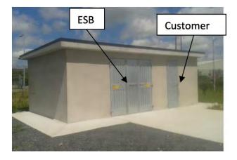
Figure 5-64 Example of MV substation
