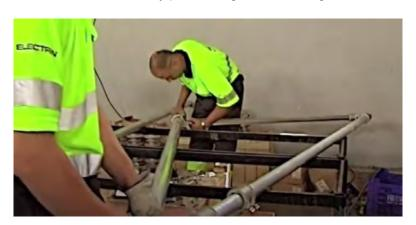
Figure 5-84 Cantilever assembly
