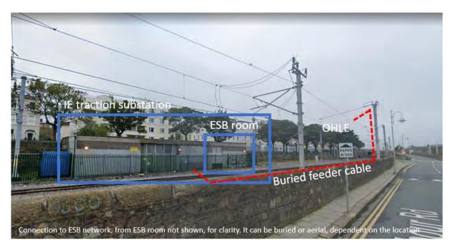
Figure 5-62 Traction substation connections
