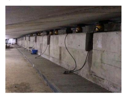
Figure 5-56 Standard bridge jacking system
