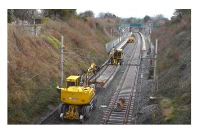
Figure 5-14 Track panel removal
