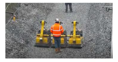
Figure 5-18 Ballast compaction
