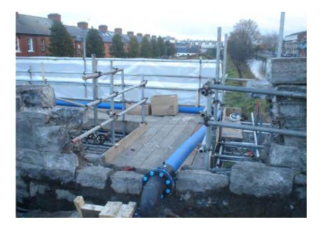
Figure 5-7 Temporary diversion along scaffolding
