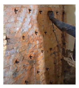
Figure 5-114 Injection of acrylic resin into vaults
