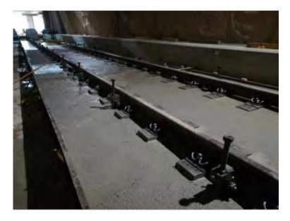
Figure 5-32 Concrete curing
