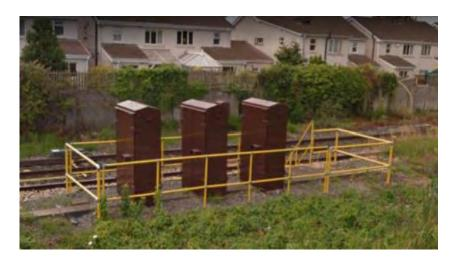
Figure 5-69 Example of three LOCs
