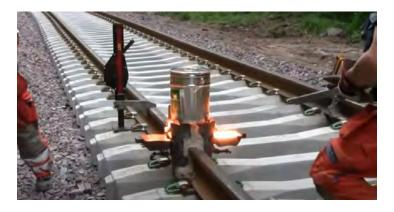
Figure 5-23 Rail joint welding
