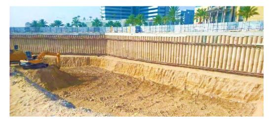
Figure 5-202 Piled wall example
