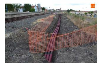
Figure 5-75 Example of buried utilities to be diverted
