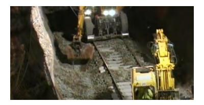
Figure 5-21 Ballast laying - second layer
