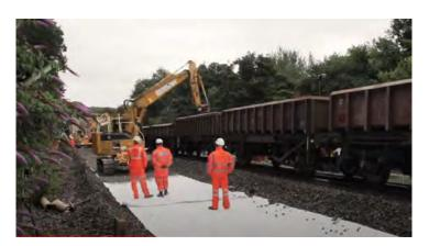
Figure 5-17 Ballast laying
