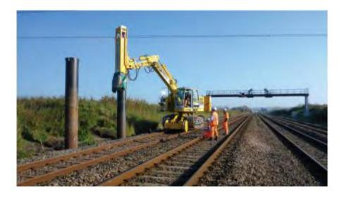
Figure 5-79 Installation of steel piles
