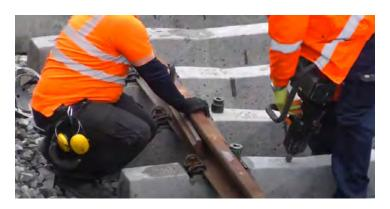
Figure 5-20 Provisional track panel joint
