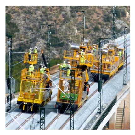
Figure 5-85 Wire installation track vehicles
