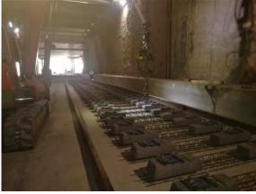
Figure 5-29 Sleeper laying on top of structural slab
