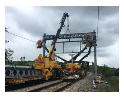
Figure 5-82 Gantry installation
