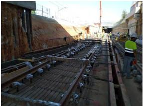
Figure 5-30 Rail and sleeper levelling
