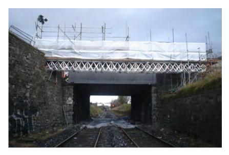
Figure 5-6 Scaffolding for temporary diversion
