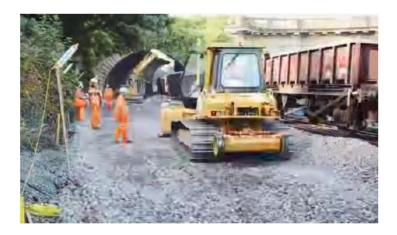
Figure 5-25 Ballast laying and compaction
