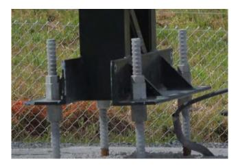
Figure 5-83 Foundation anchor for masts
